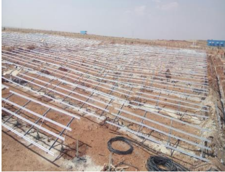
Mounting Structure Table Arrays
